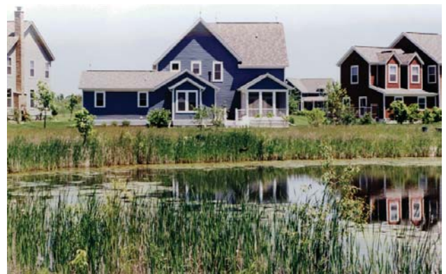
Prairie Crossing's naturalized detention basins clean stormwater and provide habitat and aesthetics.
